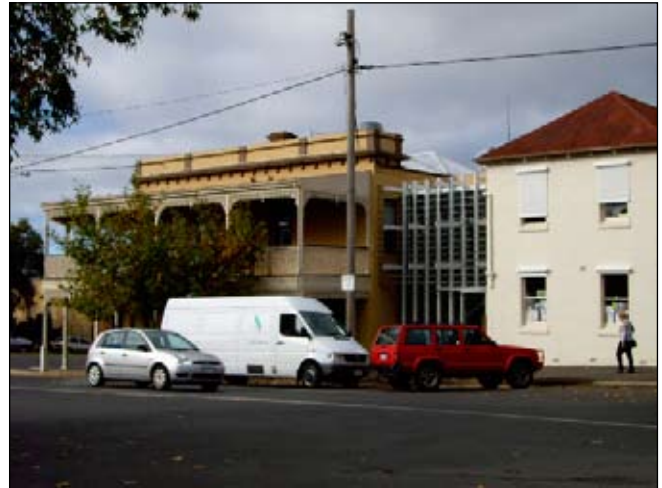
The Hub is the white building at the right of the picture
