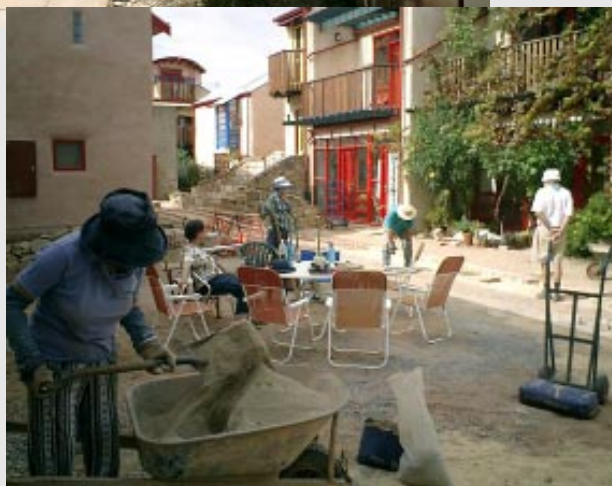
Time for a break as community members work on paving
