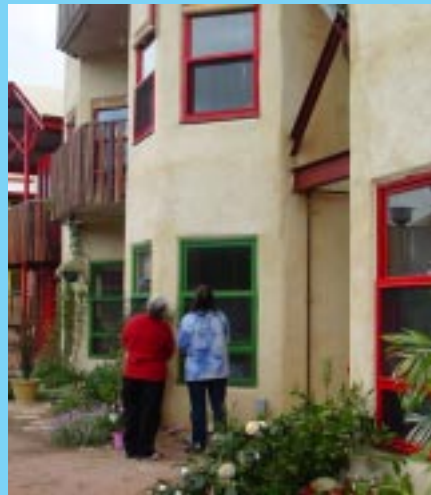
Stage 2 apartments completed in January
