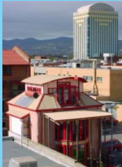
Strawbale house in Stage 2 - from the roof garden
